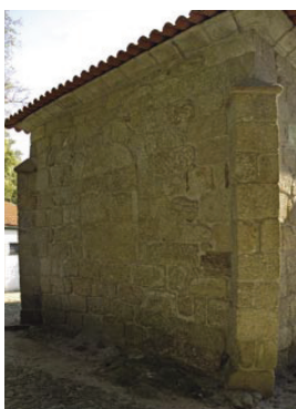
6. Transept. The angles' buttresses are usual in constructions from the late 15 th and early 16 th century.
