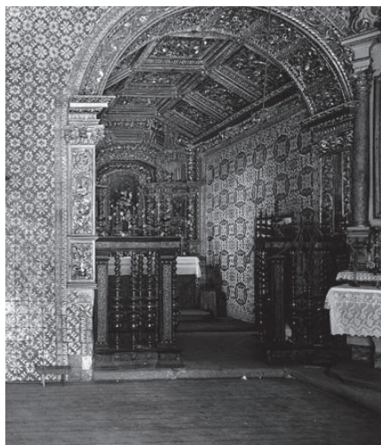
14. Chapel of Our Lady of the Rosary before restoration.
