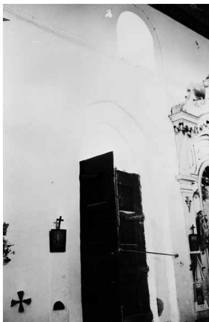
Nave. North wall. Old portal before the intervention carried out by the DGEMN. Source: IHRU archive.
