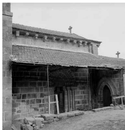
General view of the porch before the intervention carried out by the DGEMN (1960). Source: IHRU archive.
