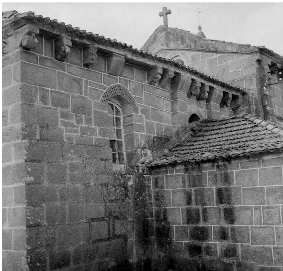
North façade. Chancel after the intervention carried out by the DGEMN (1977). Source: IHRU archive.
