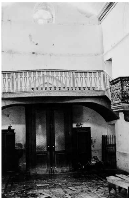
Nave. High choir before the intervention carried out by the DGEMN. Source: IHRU archive.
